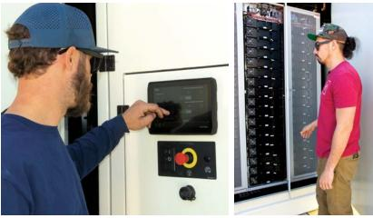
A Cat Master Microgrid Controller (MMC) acts as the brain of the microgrid, integrating the photovoltaic system, generator set, and energy storage system to maximize penetration from renewable energy sources and enhance system reliability.
